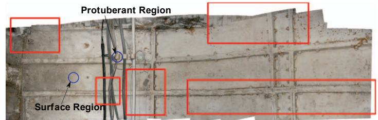
Fig. 1: The result from a state of the art mosaicing method based on the planar motion model [12]. The parallel lines (tunnel ridges) diverging along the horizontal axis of the image and mis-registrations due to protuberance are evident (within the red box).
